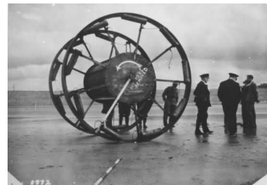
The Great Flaming Panjandrum, designed to clear beach obstacles.
