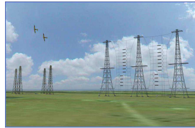
Chain Home transmitters on the left and receivers on the right.
