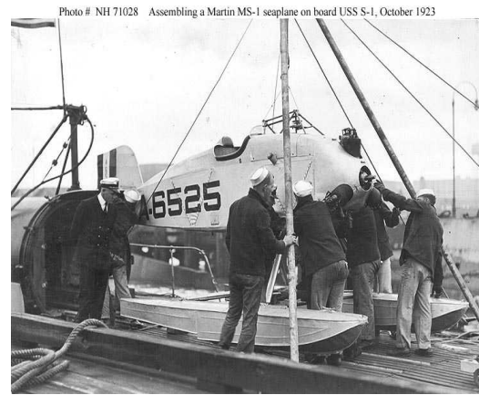
Photo # NH 71028 Assembling a Martin MS-1 seaplane on board USS S-1, October 1923
