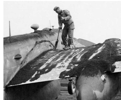
Ash deposits and damaged elevators on 240th B-25s
